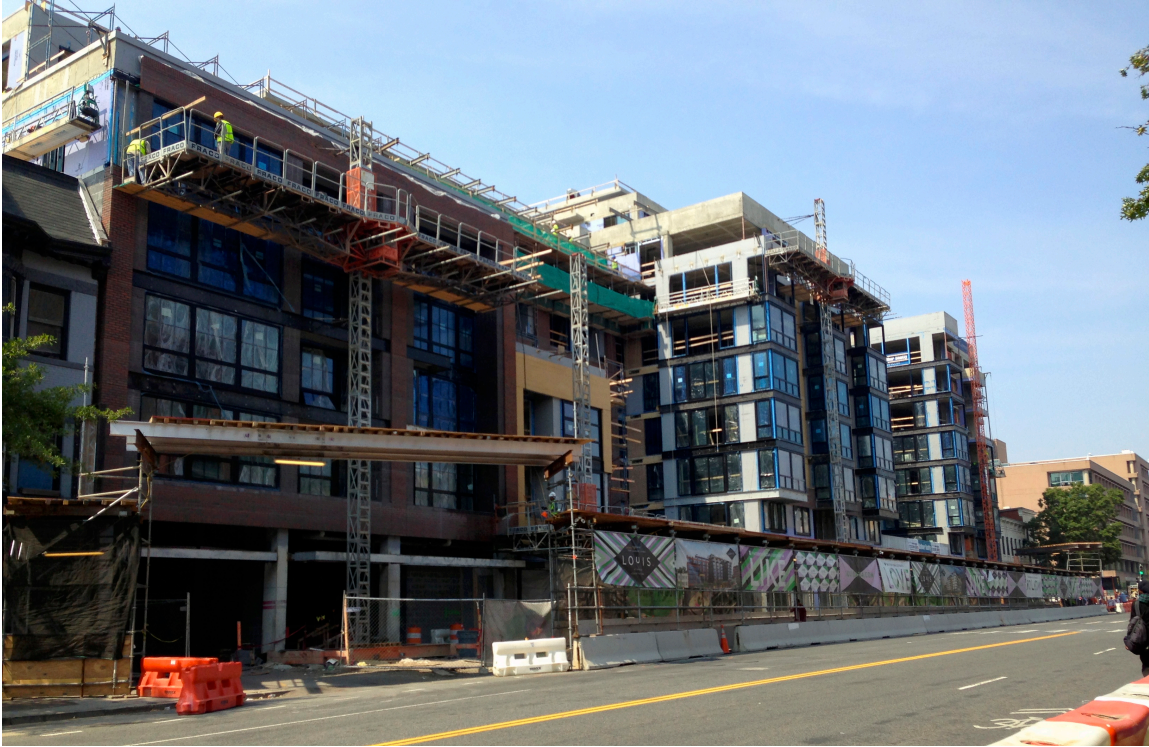
Above is a view of the actual project from 14 th Street portraying the obstruction onto the public sidewalk requiring signage and protection as appropriate for the ongoing construction. (picture by Russell Voigt)
