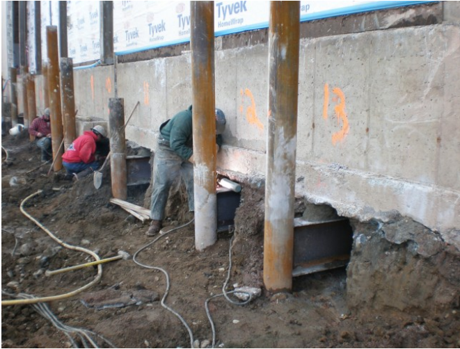
An example of underpinning by bracket piles utilized for the adjacent post office building to the south in the actual construction and will likely be needed for the nine-story building in the adjacent northwest corner for the proposed redesign. Photo by moretrench.com
