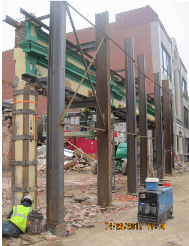
Historic Façade support perspective. Photo by Balfour Beatty Construction
